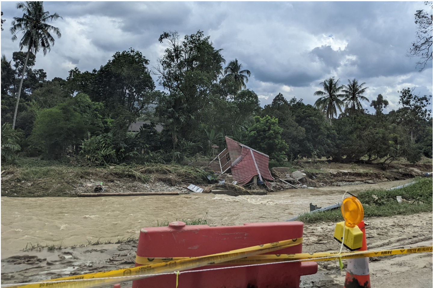
Figure 19: A house is destroyed near Sungai Langat in the week after heavy rains that caused the massive 2021 flood in Hulu Langat, Selangor. Source: Jehan Wan Aziz.
